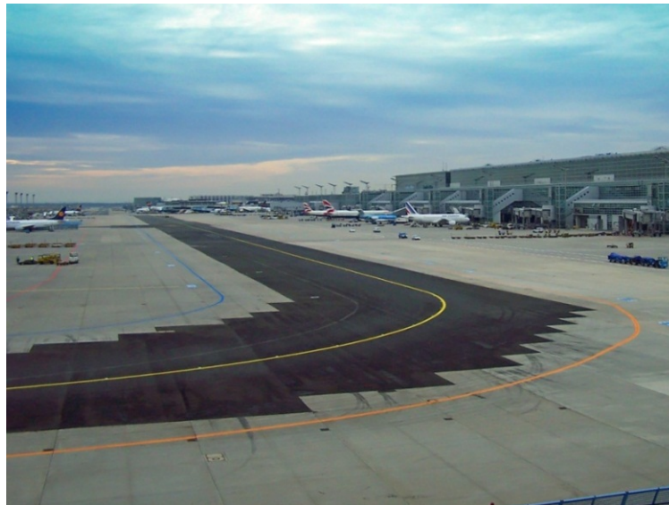
Figure 12: APTR at Frankfurt airport
